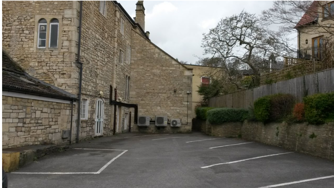
Rear of Manvers House from car park
