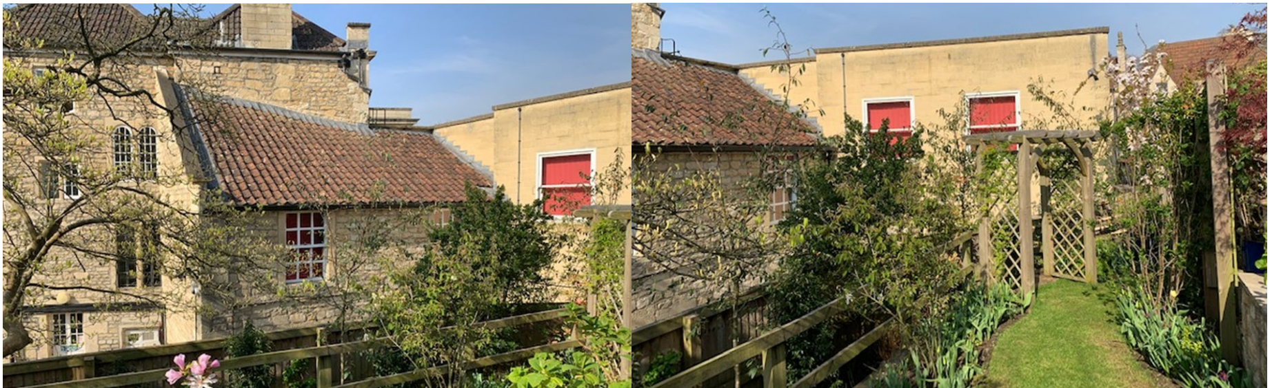
Rear No. 6 Mill Lane looking towards rear of Main Block and NE elevation
