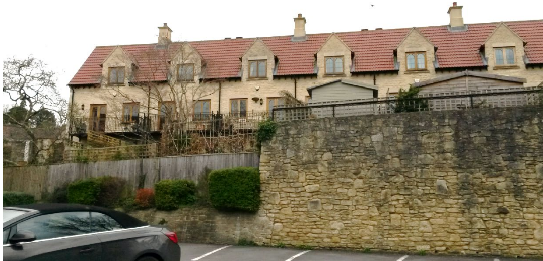
Rear of 1-6 Mill Lane
