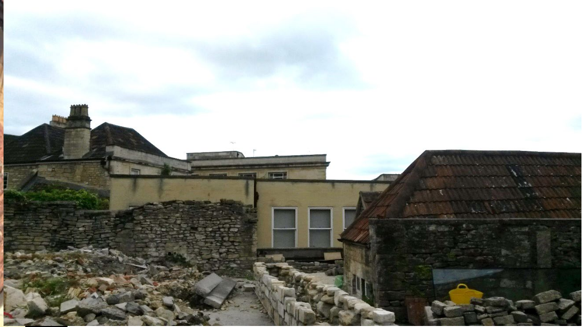
View of rear of North Block from No. 24 Silver Street
